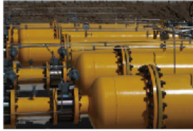
▲ Municipal Engineering & Utilities
